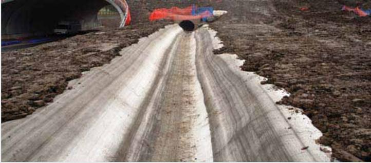
CC can be rapidly unrolled to form ditch or tank lining. It is significantly quicker and less expensive to install than conventional concrete ditch lining. It will conform to a range of ditch profiles and curves and requires no specialist plant equipment. The 30m ditch shown above was lined in 45min.
