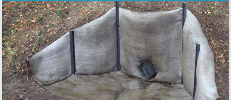
CC can be used as an effective and faster alternative to precast or cast-in-place concrete culverts.
