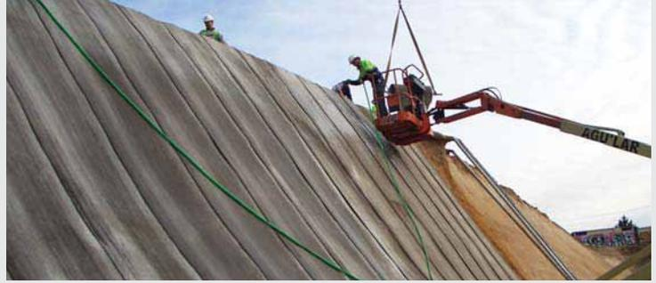
CC can be used in erosion control applications such as temporary and permanent slope protection, retaining walls, boulder fences, low level bunds and river bank and dam revetments.
