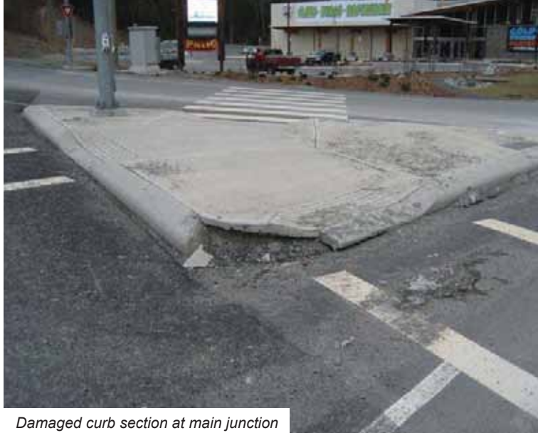
Damaged curb section at main junction
