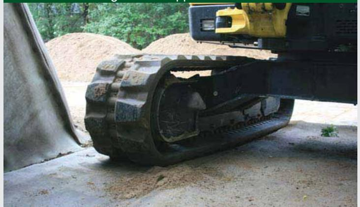
CC can be secured with ground anchors to create a concrete surface. CC4 can be used for dust suppression and the thicker CC8 and CC13 for helicopter landing areas and track surfacing.
