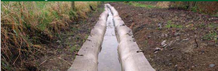
CC can be unrolled rapidly to form a hardened, water proof concrete ditch or tank. It will conform to a range of ditch profiles and curves and requires no specialist plant equipment. Joints can be sealed to withstand over 3m of water pressure.
