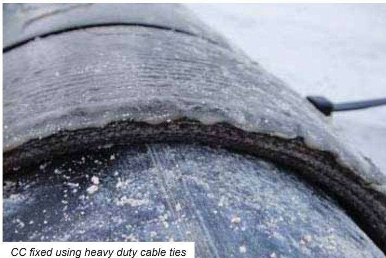
Completed CC pipeline protection
