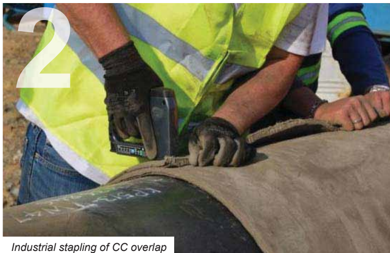
2m circumference PVC coated multi-purpose fuel/oil pipeline
