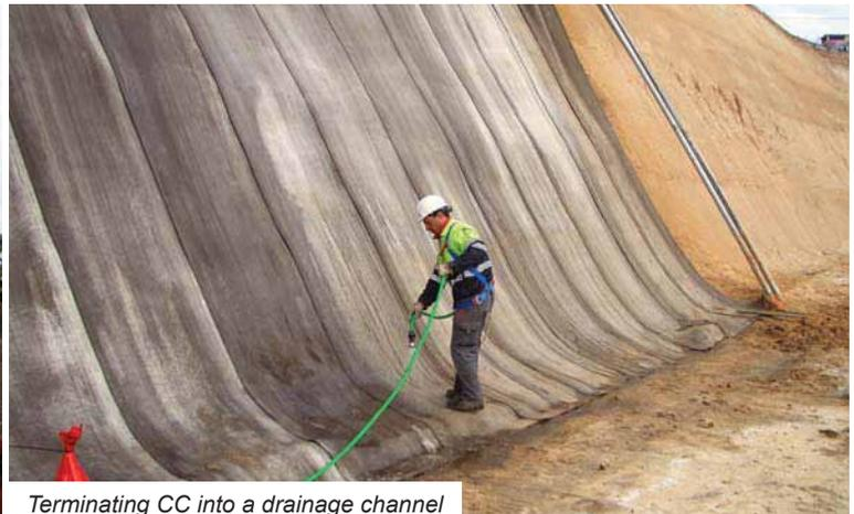
Terminating CC into a drainage channel
